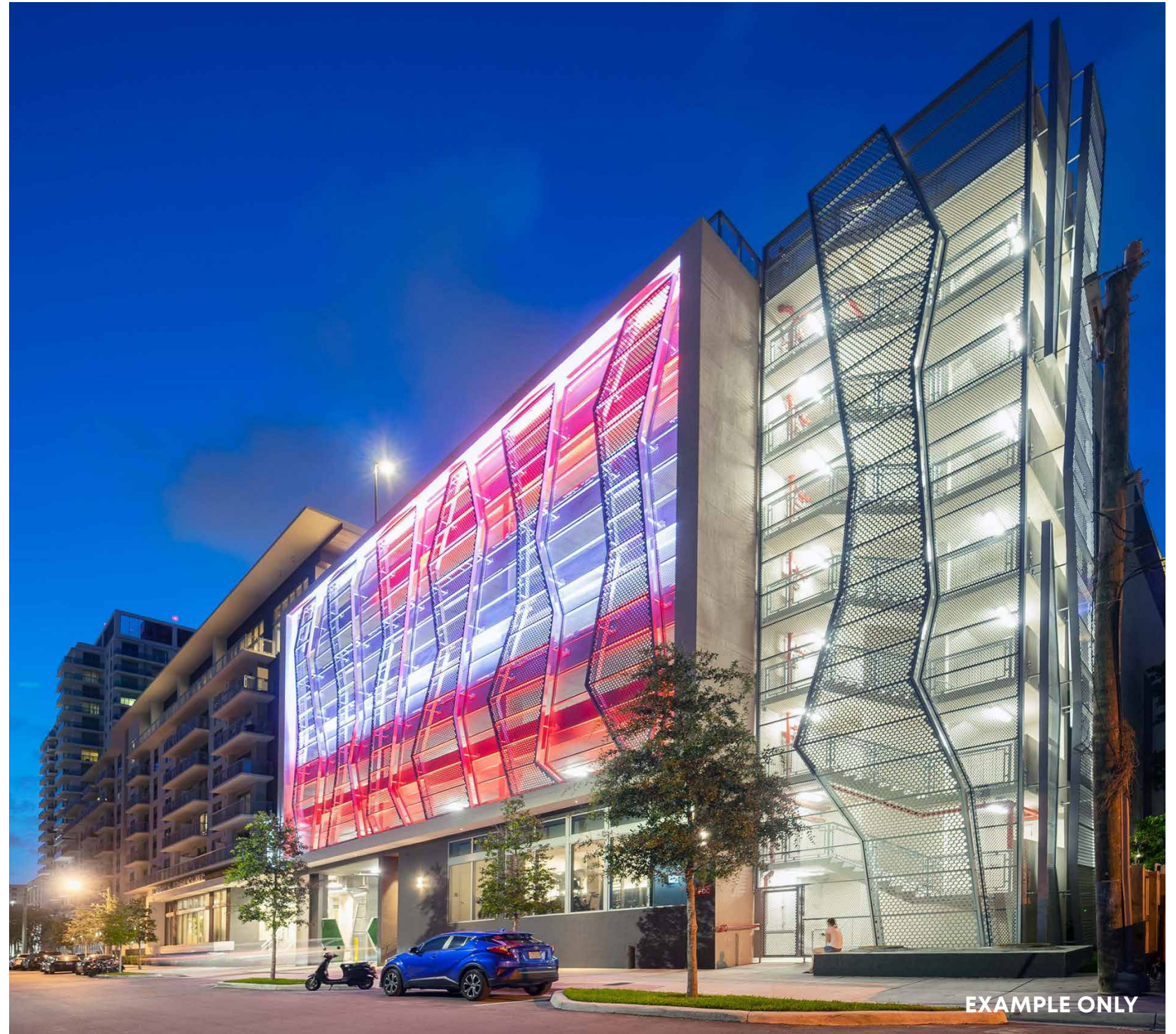
FACE AND BACKLIT LIGHTING EXAMPLE PHOTO - PERFORATED PANELS ILLUMINATED FROM EXTERIOR AND INTERIOR LIGHTING
