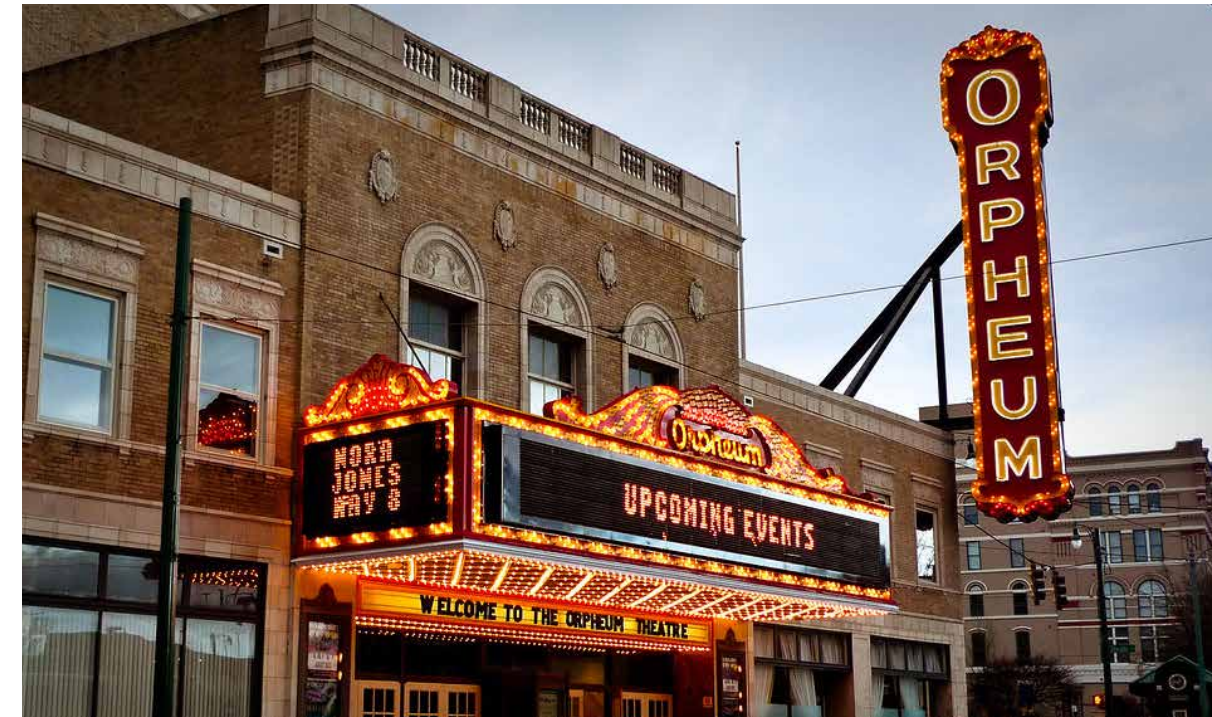
ORPHEUM THEATRE - MARQUEE CANOPY
