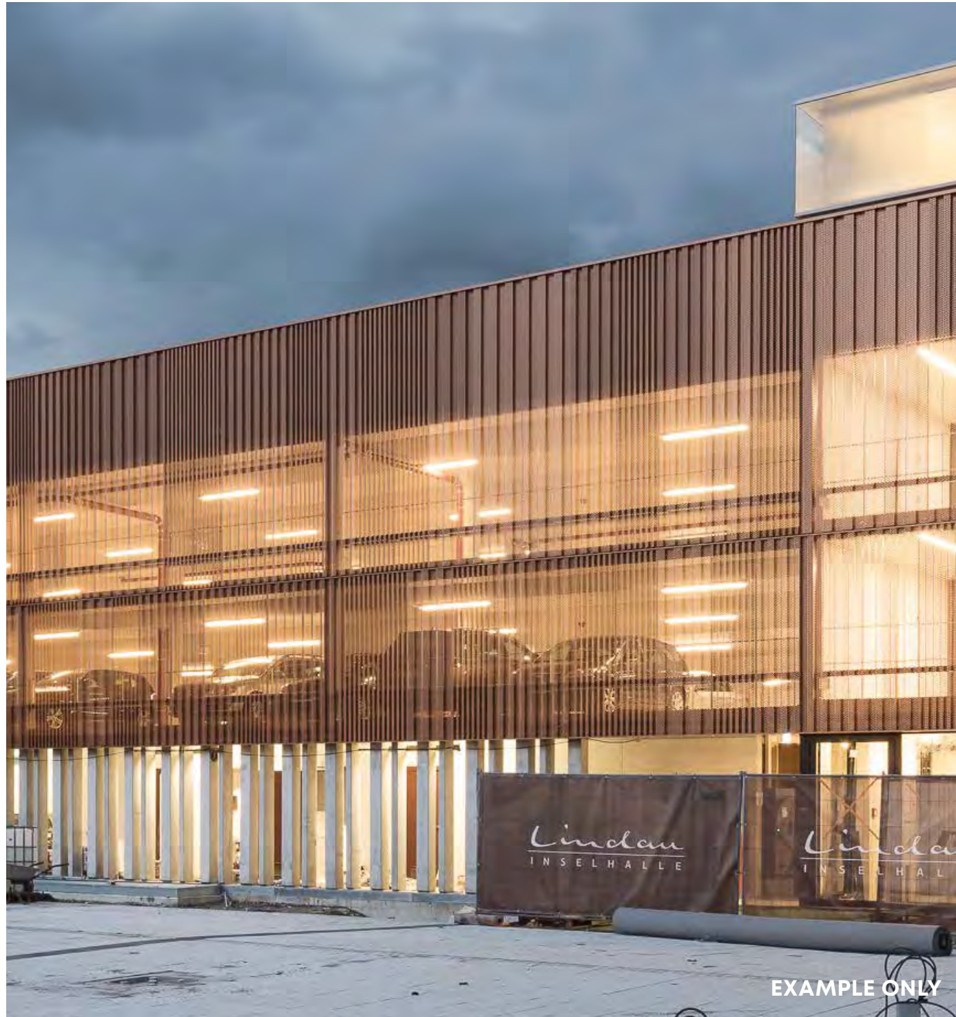
BACKLIT LIGHTING EXAMPLE PHOTO - PERFORATED PANELS ILLUMINATED FROM GENERAL PARKING LIGHTING
