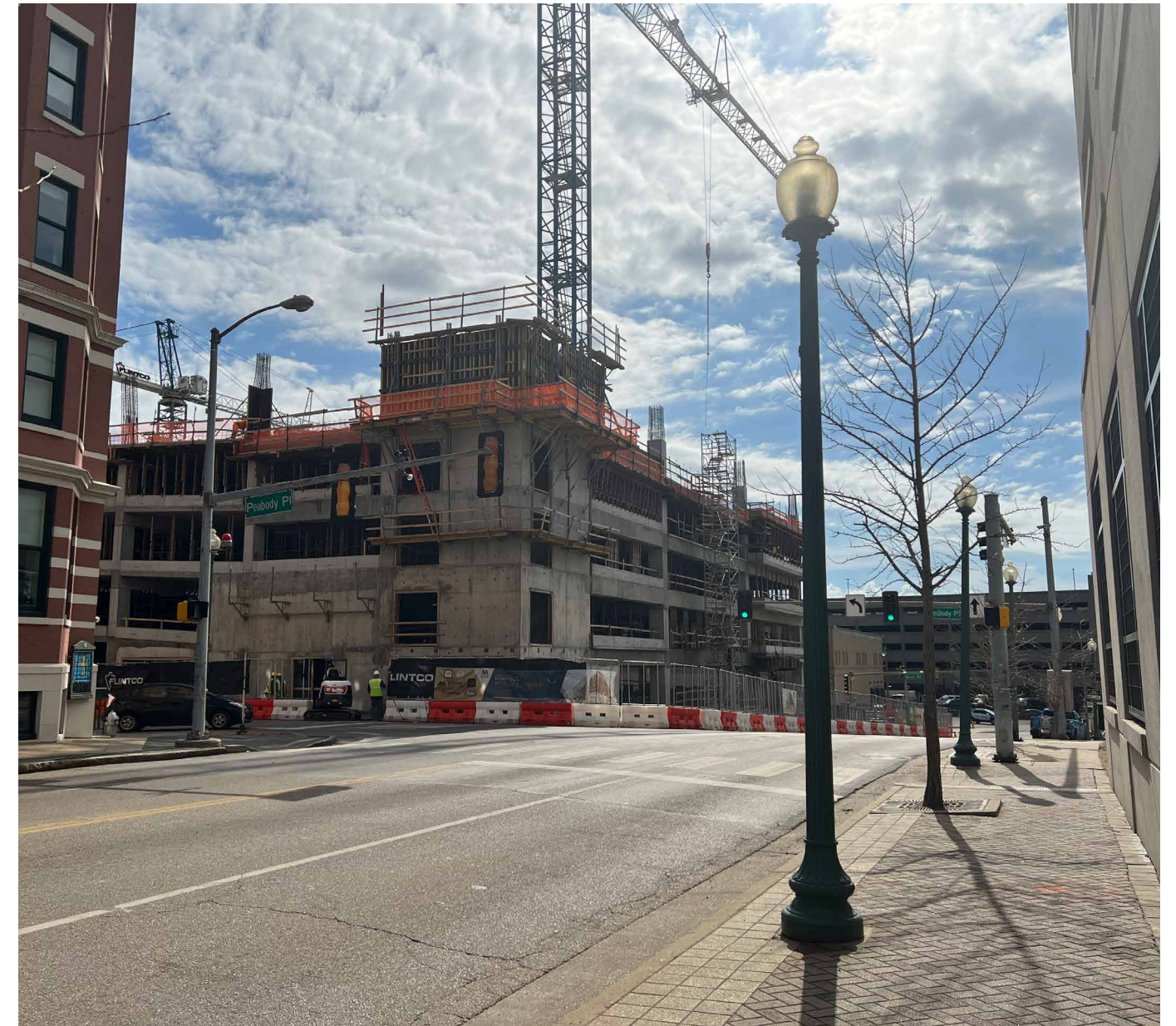
FRONT STREET AND PEABODY PLACE INTERSECTION - VIEW TO MOBILITY CENTER
