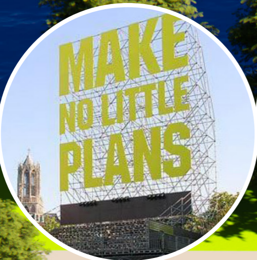
STAGGERED SCAFFOLDING INSTALLATION FEATURING AN EVOCATIVE PHRASE
