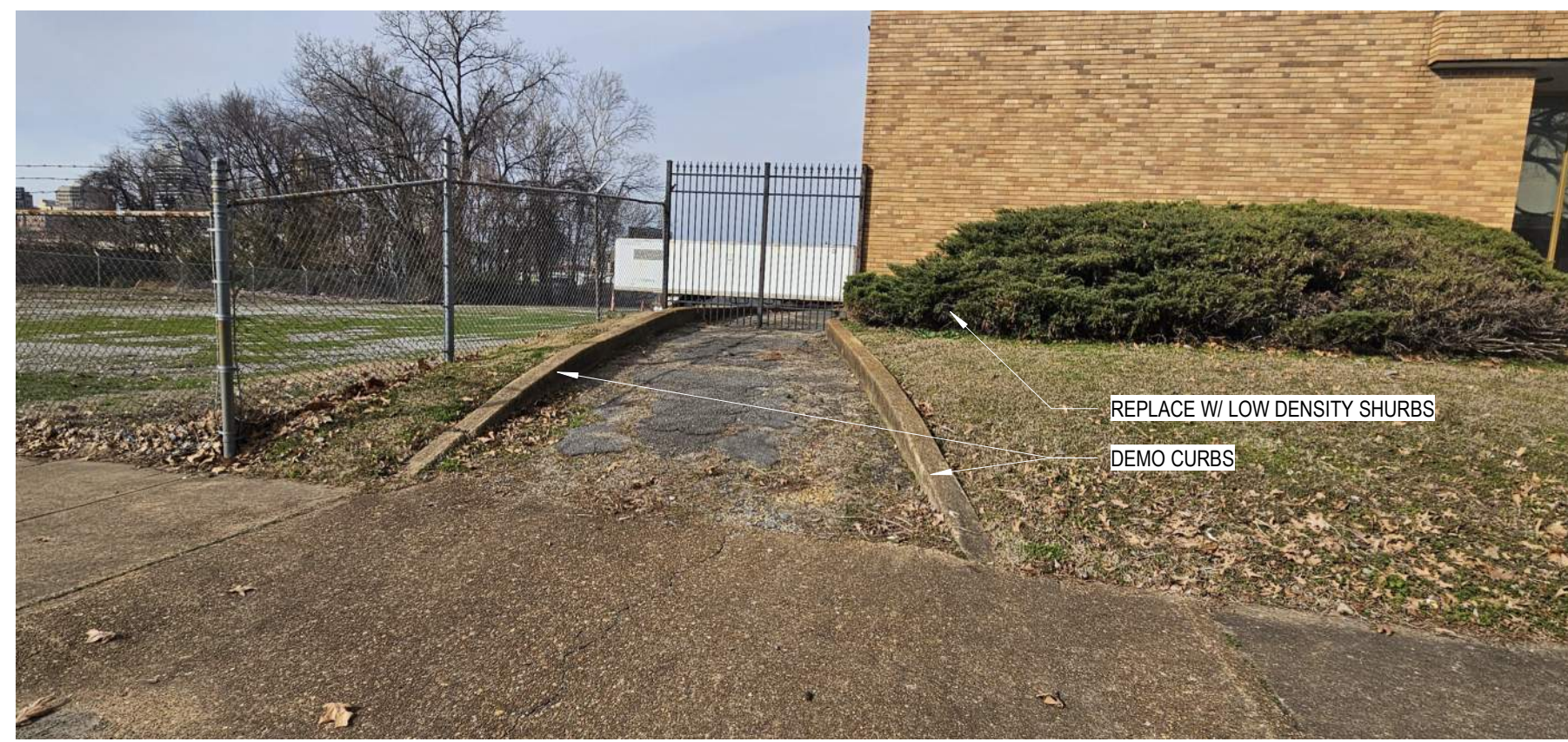
VIEW FACING NORTH
