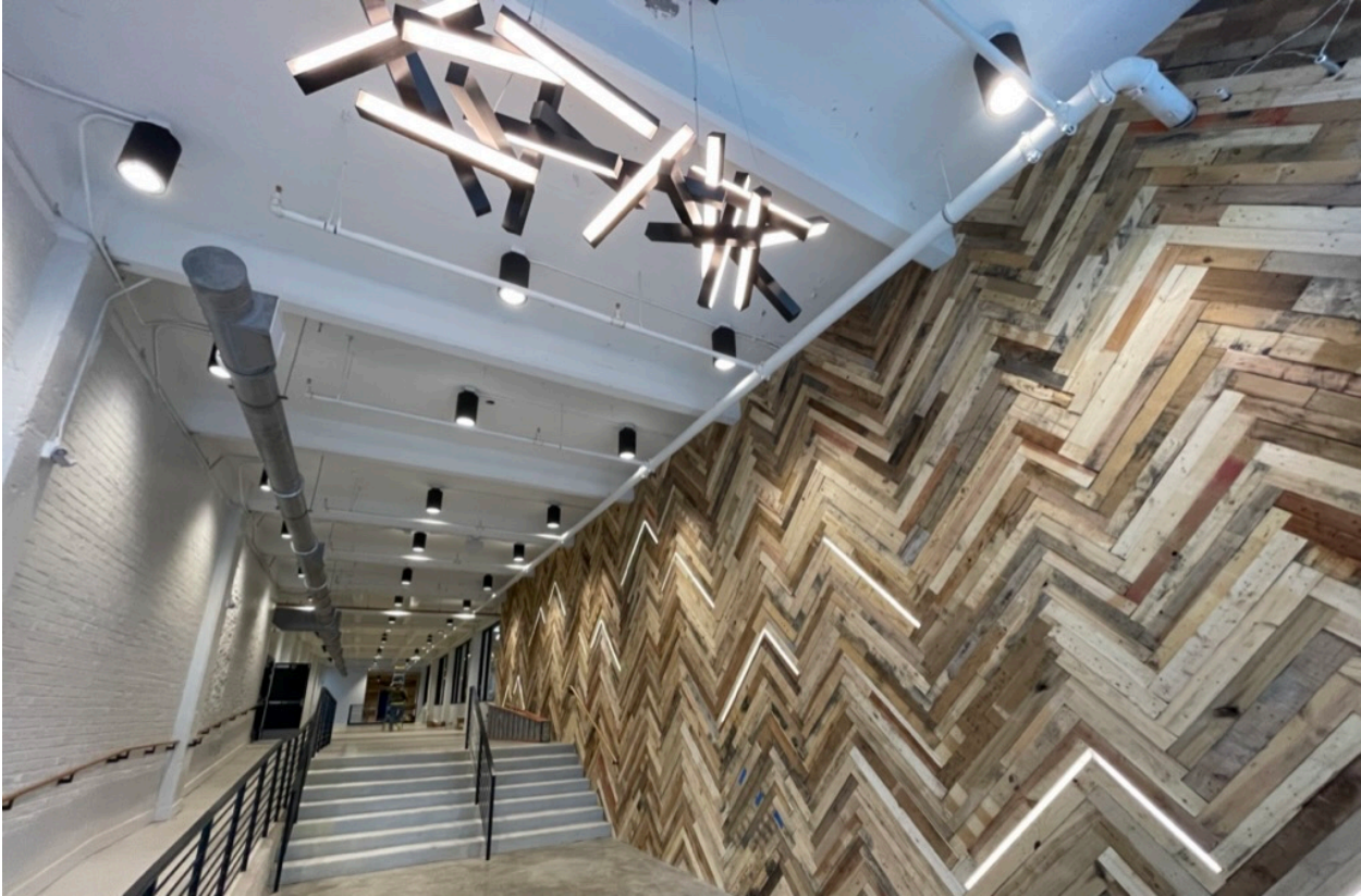
Memphis Made Brewery Interior (Under Construction)
