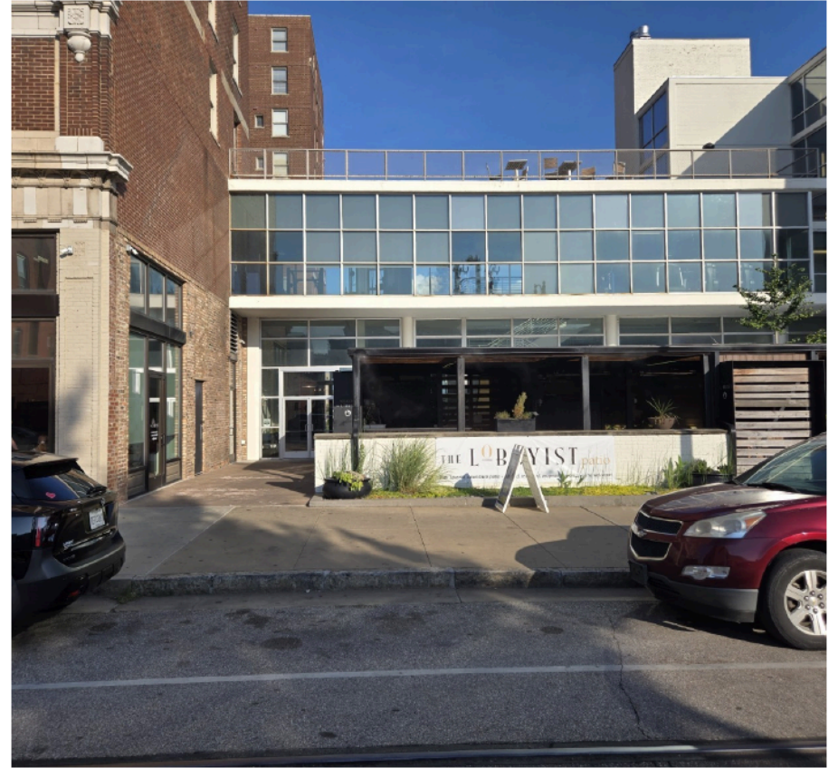
South Main frontage / patio enclosure
