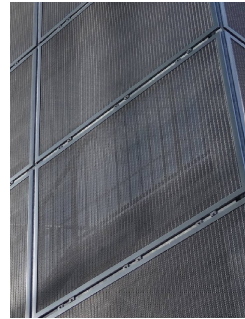
MP-1: METAL MESH SCREEN PANEL - GRAY
