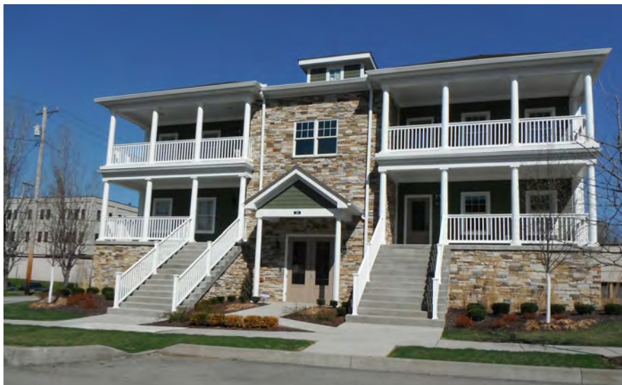
Mansion apartment building
