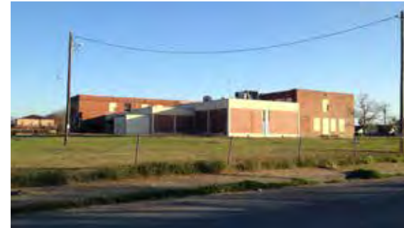
The former Crossley Elementary School building, damaged by a 2013 fire
