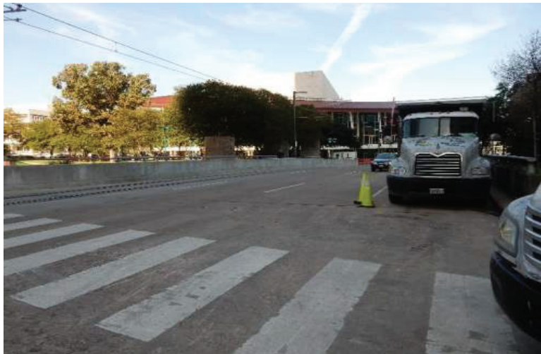
Figure A.13 Roadway Looking West
