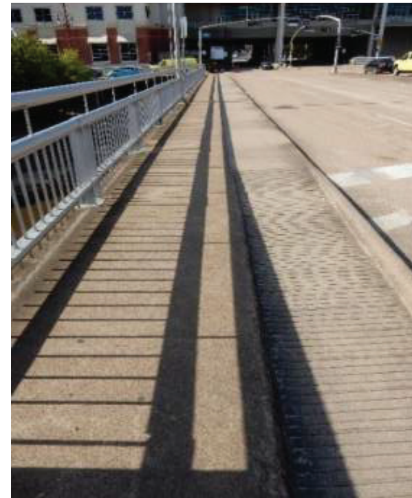
Figure A.06 East Sidewalk Looking South
