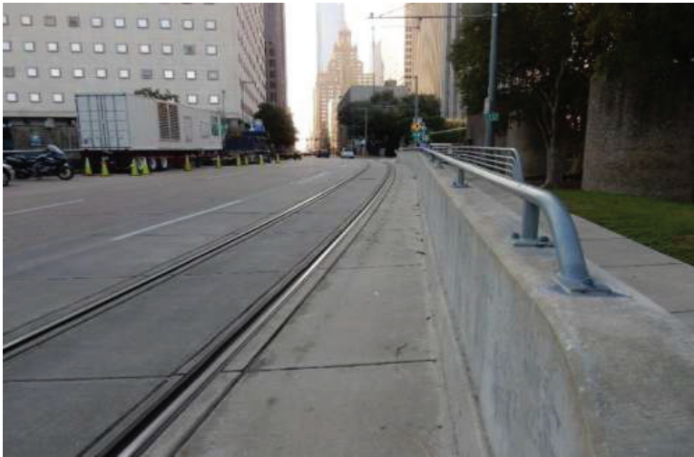
Figure A.12 Roadway Looking East
