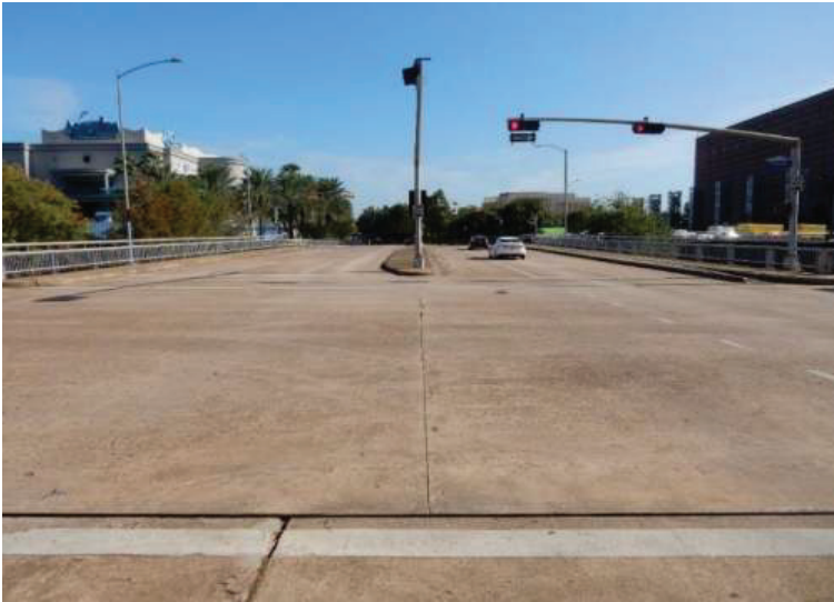
Figure A.04 Roadway Over Bridge Looking North
