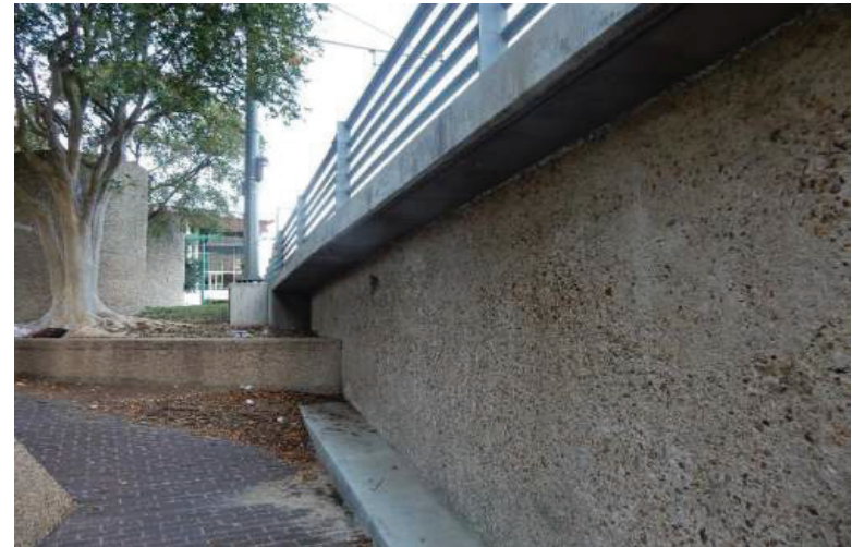
Figure A.19 Retrofitted South Sidewalk Overhanging Wall
