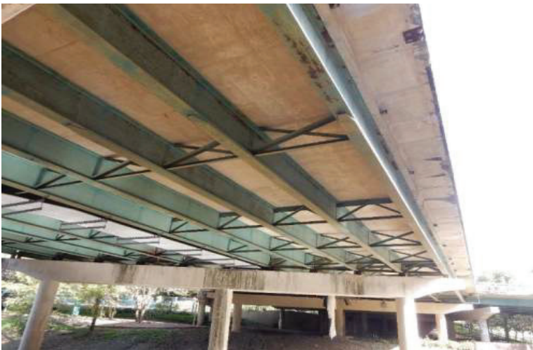
Figure A.05 Superstructure & Substructure Looking North
