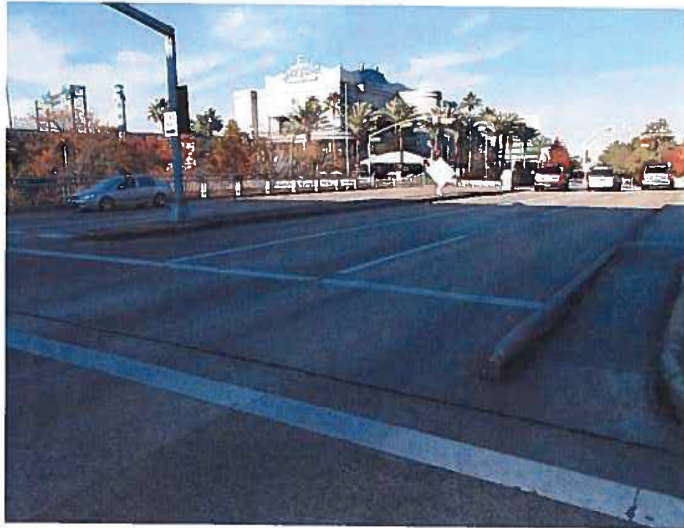
Roadway Over Bridge
