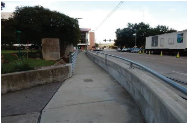
Figure A.18 South Sidewalk Looking West
