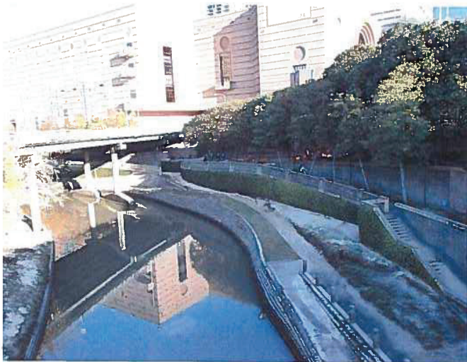
Downstream View From Bridge
