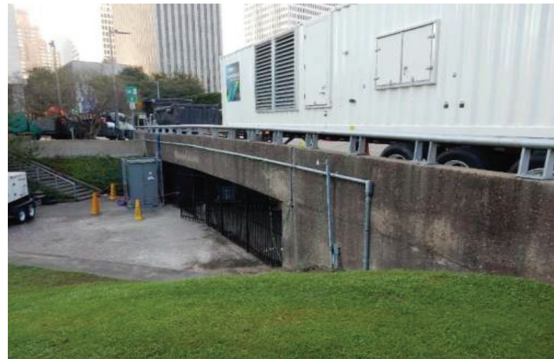
Figure A.14 Elevation Looking Southeast
