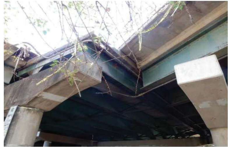
Figure A.10 North Bridge Transition
