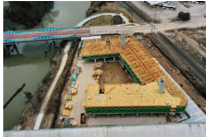
McKee City Living under construction
