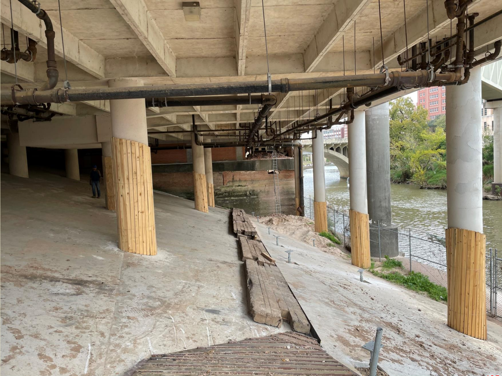
View underneath IPC Building
