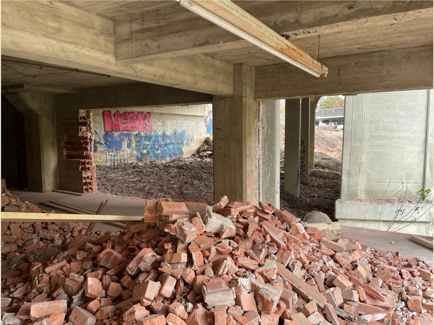
Demolition in the Wilson Building
