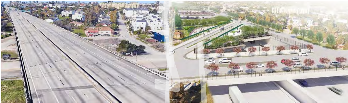
IH-60 at Alameda "Before"
