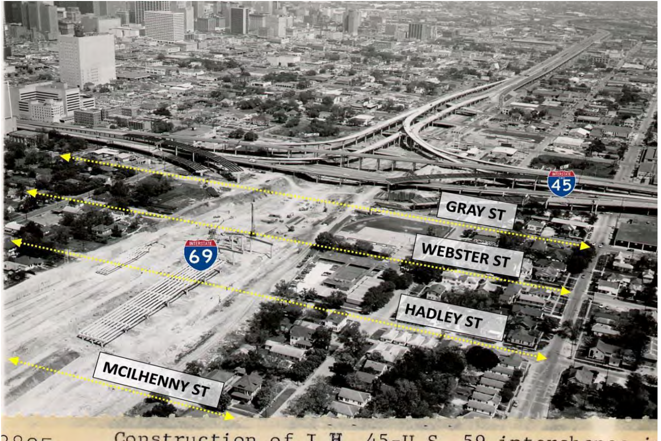
2005 Construction of I-45-I-69 interchange 1972 Demolition/destruction of Third Ward urban fabric to accommodate I-69
