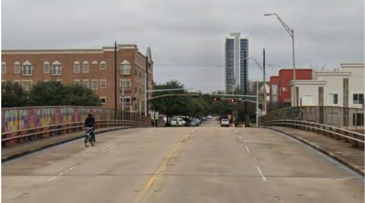
Existing Tuam St Bridge over I-69
