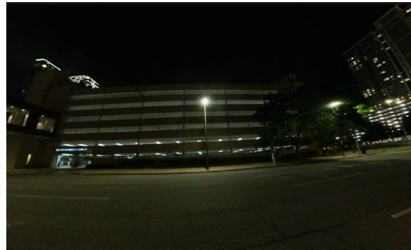
Large amounts of both garage parking and surface parking lots leads to disconnects between the areas with high hospitality locations. Surface parking lots are often unlit or poorly lit at night, creating dark voids next to the sidewalks.
