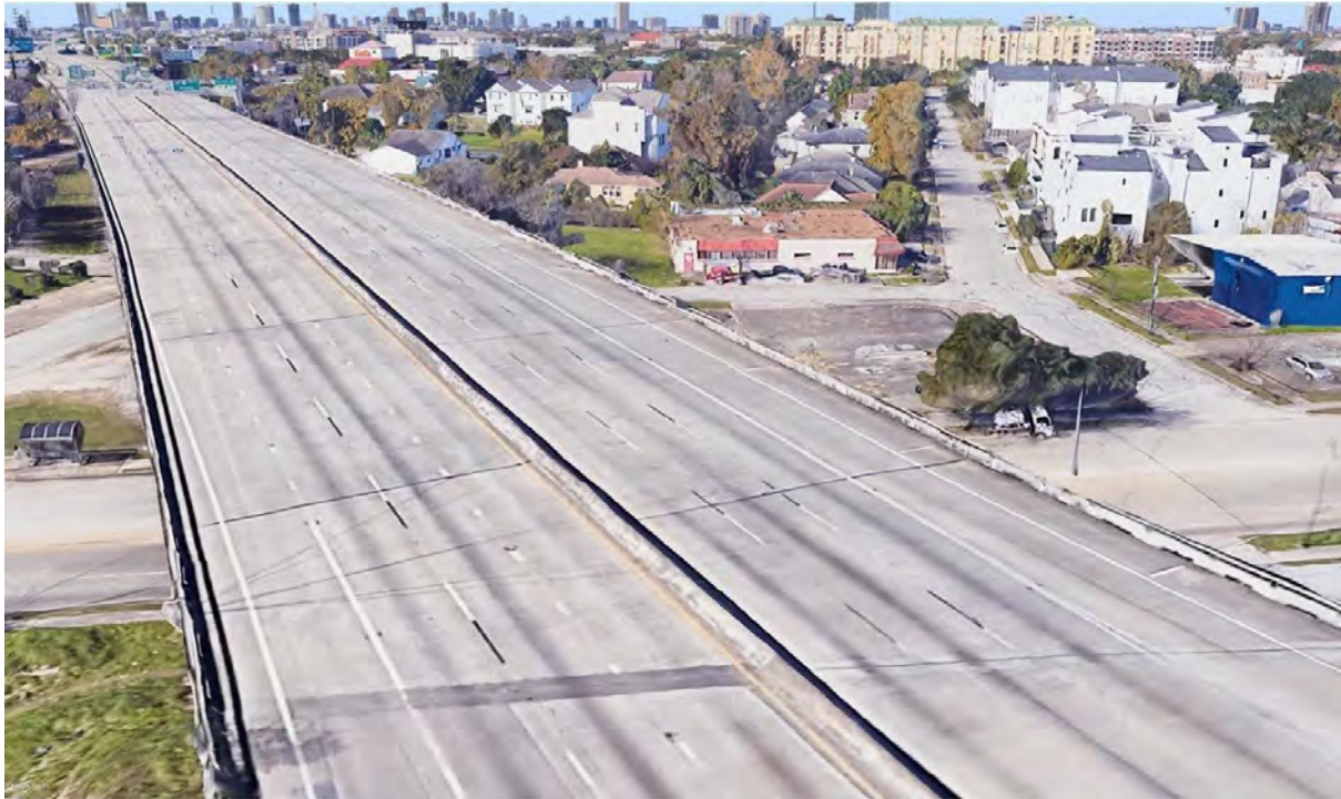
Existing elevated I-69 at Alameda Rd
