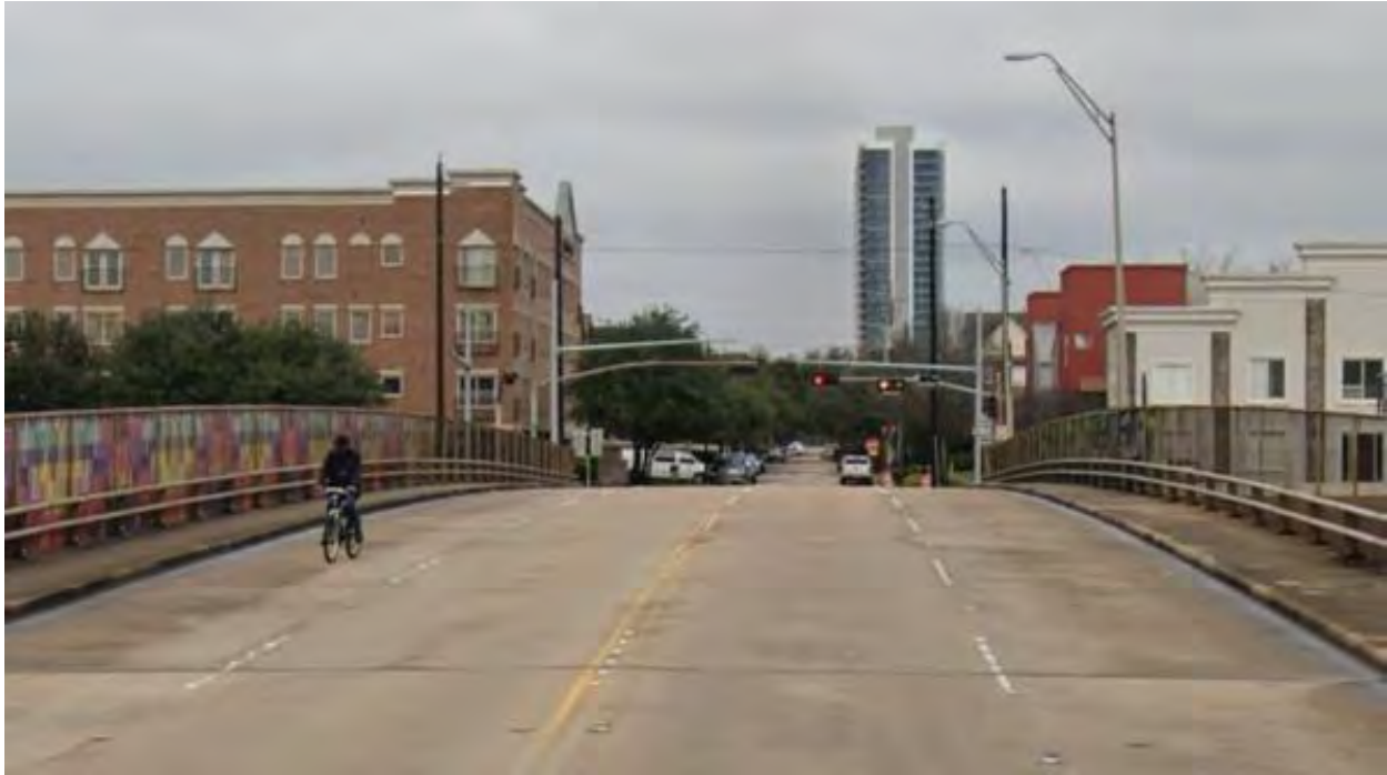
Existing Tuam St Bridge over I-69
