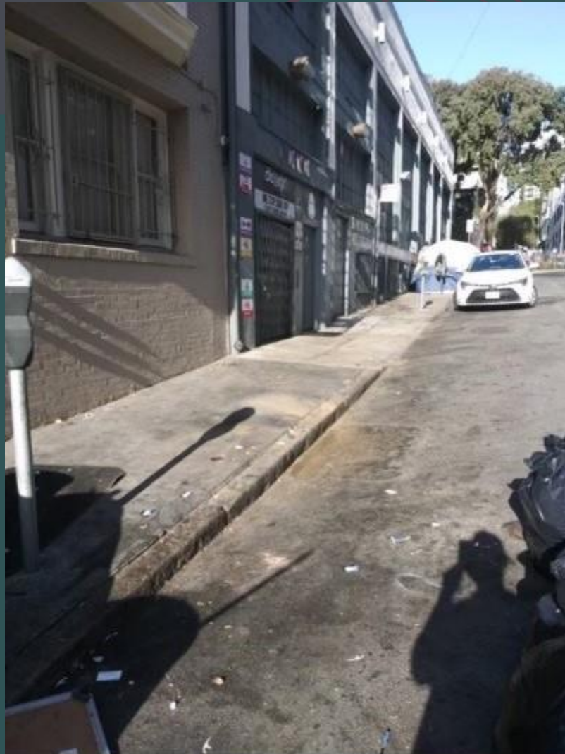
Olive Alley / After
