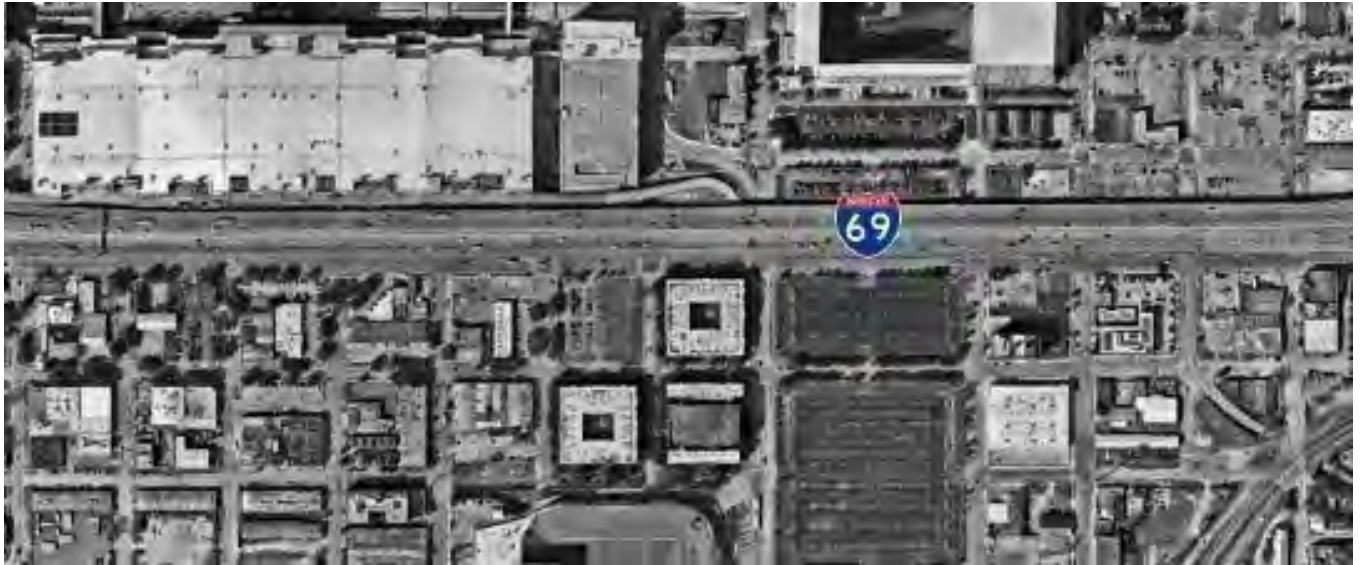
Existing highway condition at I-69 at George R Brown Convention Center
