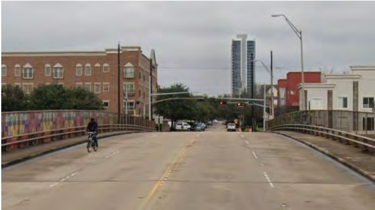
Existing Tuam St Bridge over I-69
