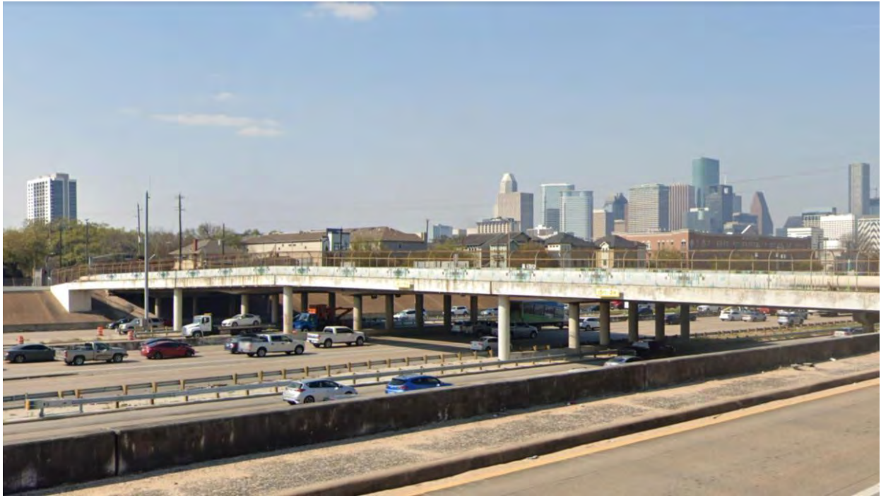
Existing Elgin St Bridge over I-69
