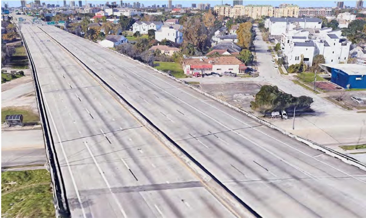
Existing elevated I-69 at Alameda Rd
