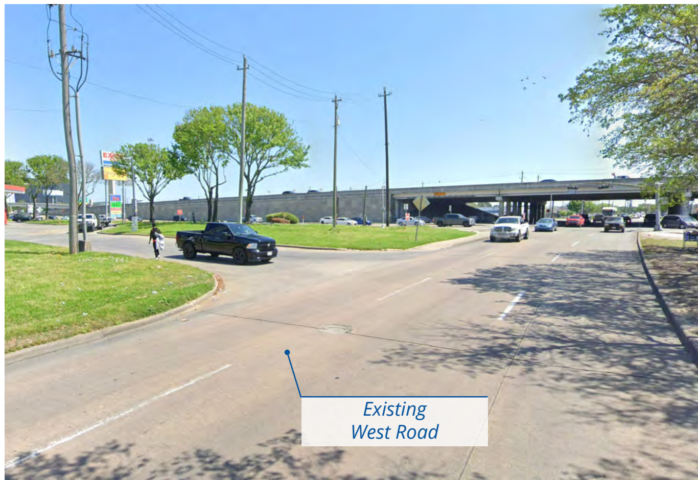
Existing I-45 and West Road
