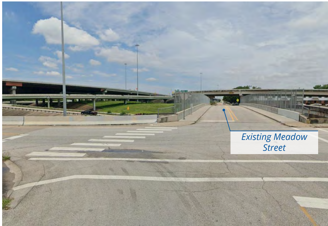
Existing I-10 and Meadow Street
