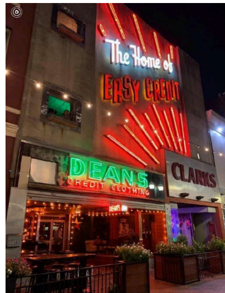
Figure 1. Past image of facade when neon signage was operational.
