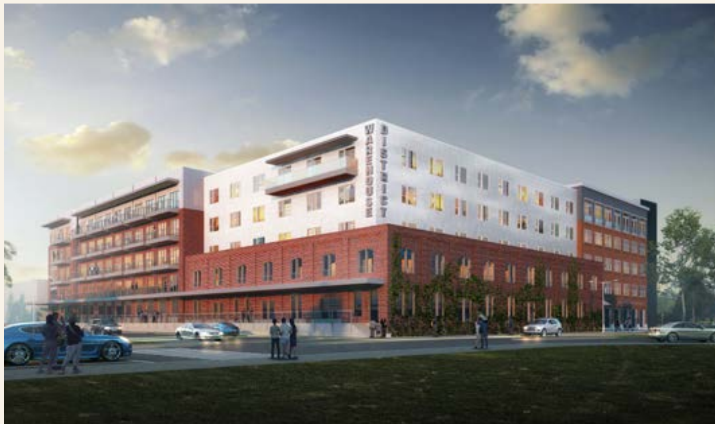
THE WAREHOUSE DISTRICT DEVELOPMENT PRE-LEASED UNITS IN DECEMBER 2023 WITH FIRST MOVE-INS SCHEDULED FOR FEBRUARY 2024.
