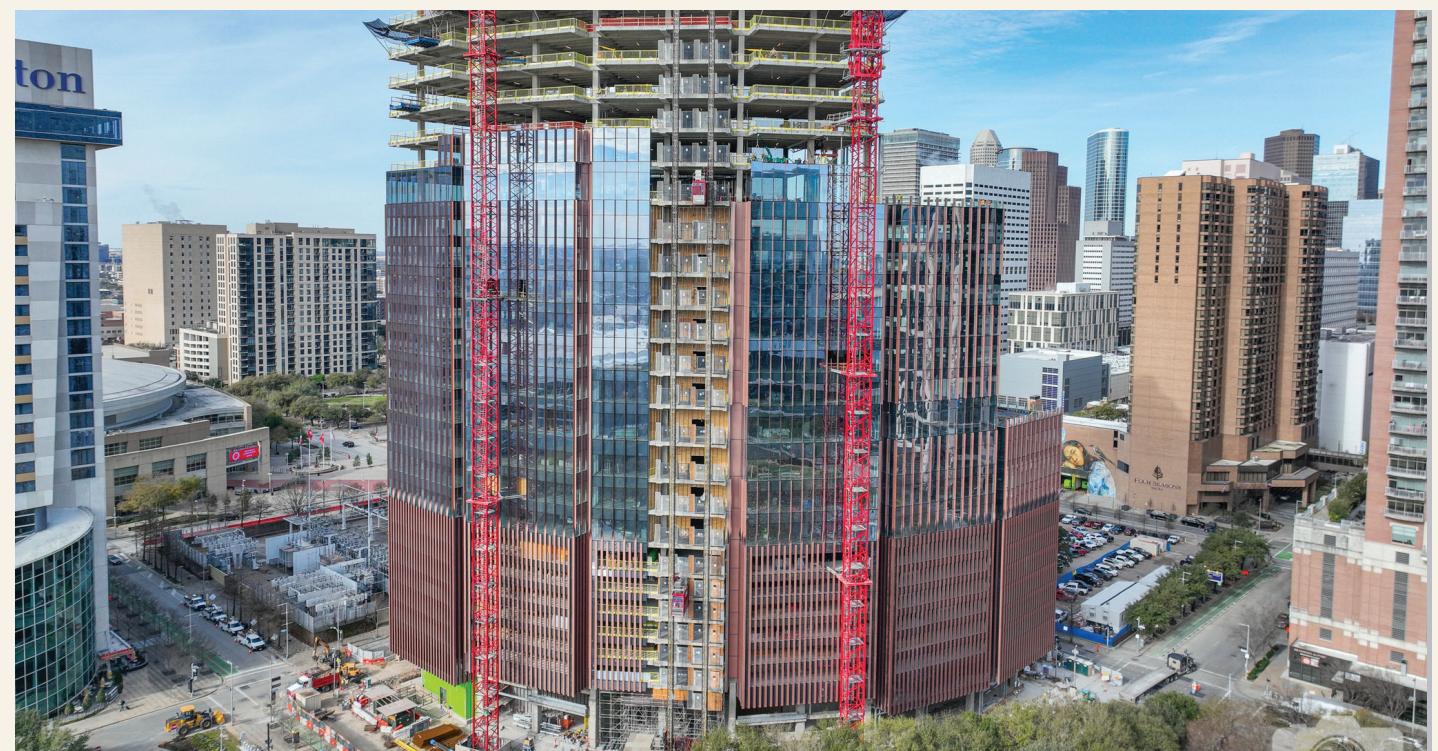
1550 ON THE GREEN UNDER CONSTRUCTION IN 2023
