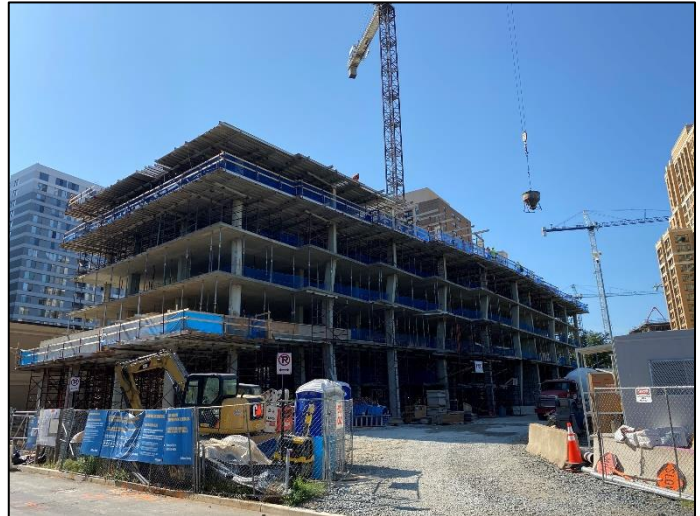
View of Site Looking Southeast – July 14th, 2021
