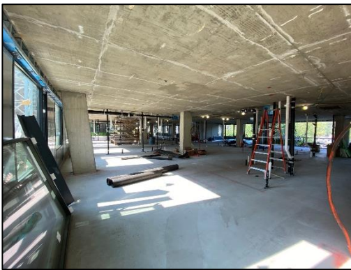
View of Window Installation on Third Floor – September 8 th , 2021
