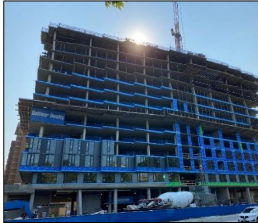
View of Site Looking East – September 13 th , 2021
