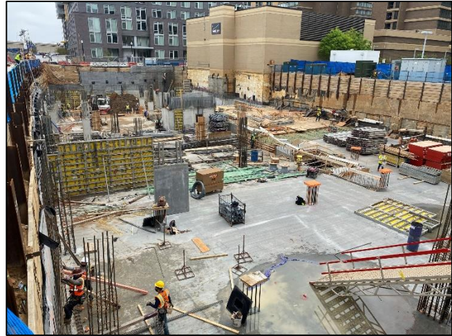
View of Site Looking Northeast – April 13, 2021
